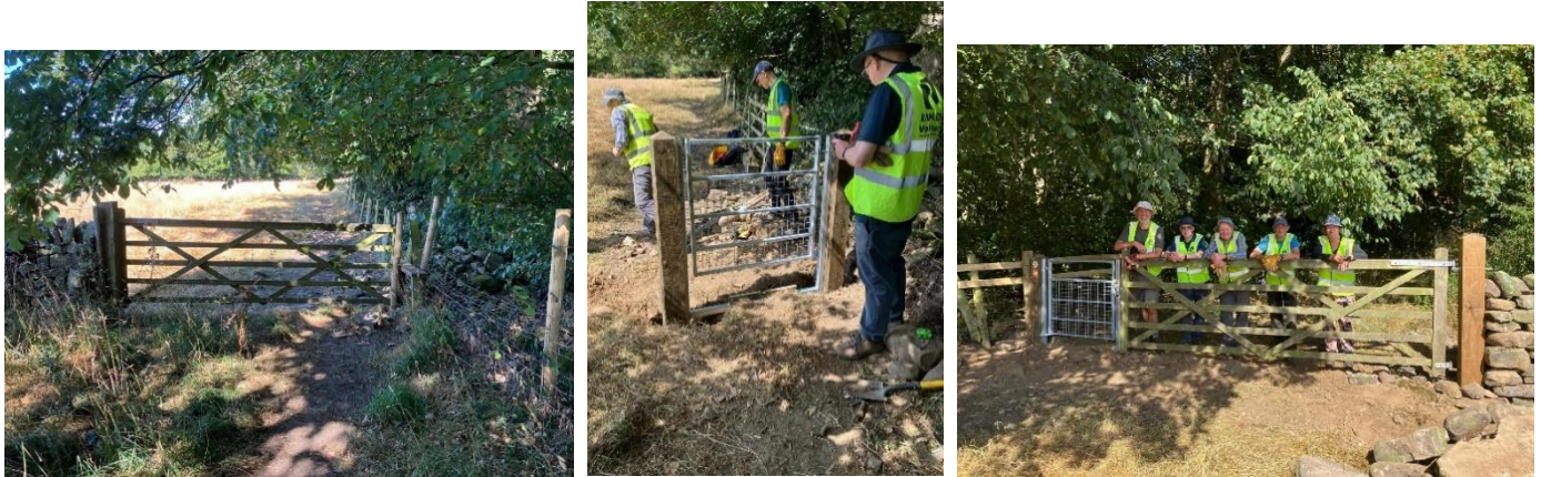
Before and after photos of gate install off Denton Rd, 10 August 2026
