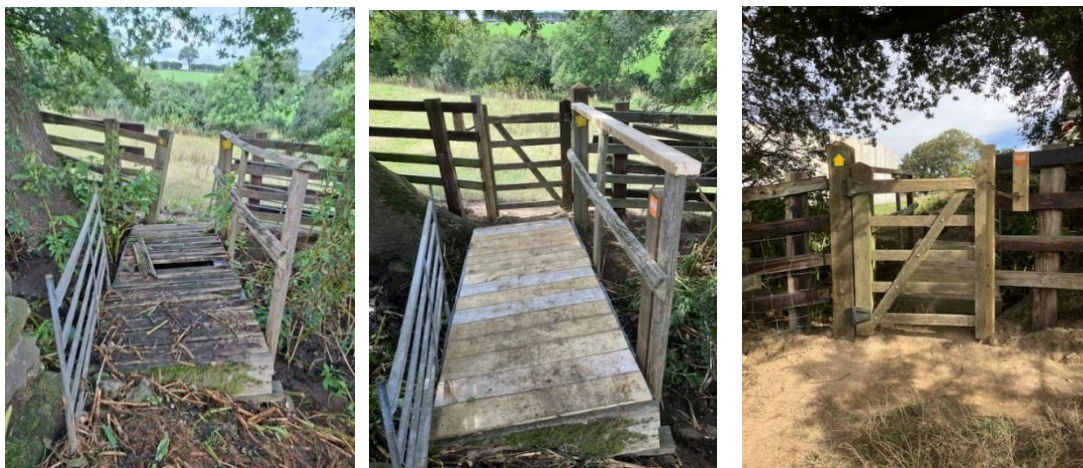
Before and after photos of bridge repair and gate reinstall, near North Rigton, 4 September 2026
